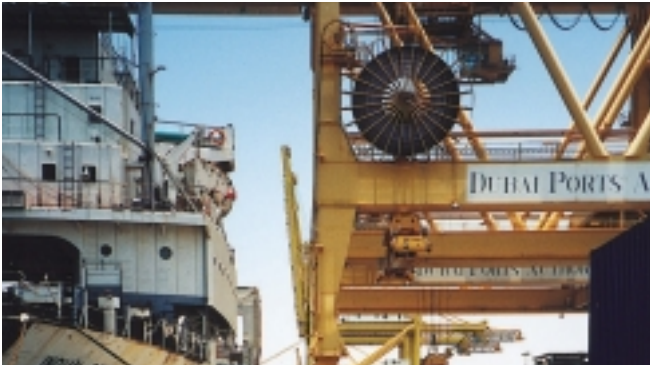
Cavotec Specimas reel in action in the Port of Dubai
