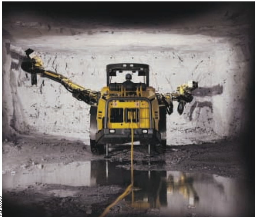
An Atlas Copco drilling rig at work in a Swedish tunneling project, equipped with a Cavotec Specimas cable reel and Cavotec Connectors.
